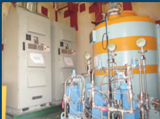
M/T George S. – DWT: 158,033 tons – Retrofit installation of BWTS (Hyundai Hi-Ballast)
